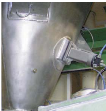
Cleaning bunker walls
